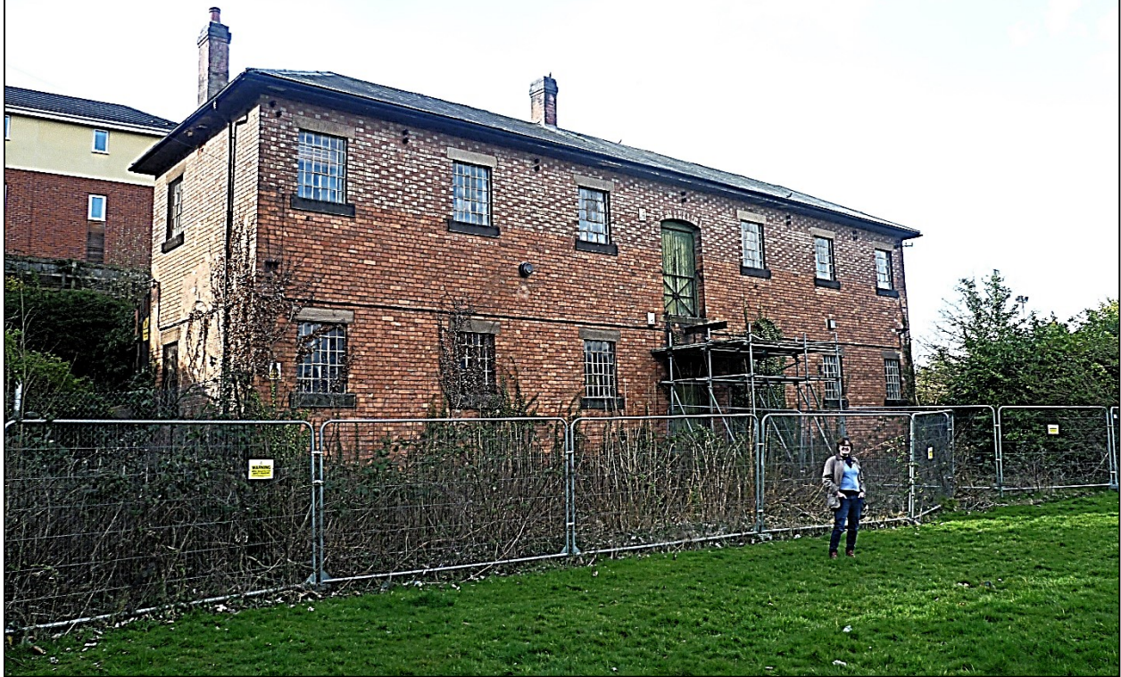
Rowditch Barracks: drill hall, looking NW with parade ground in front
